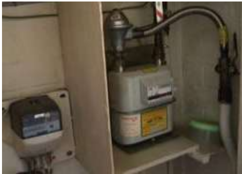
Asbestos panelling around a gas meter
