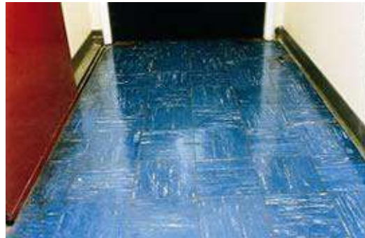
Asbestos containing floor tiles in a corridor
