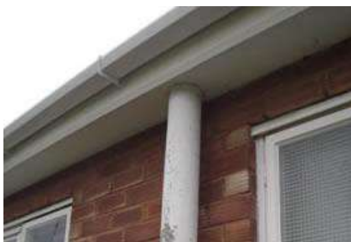
Asbestos cement drainage pipe (downpipe)
