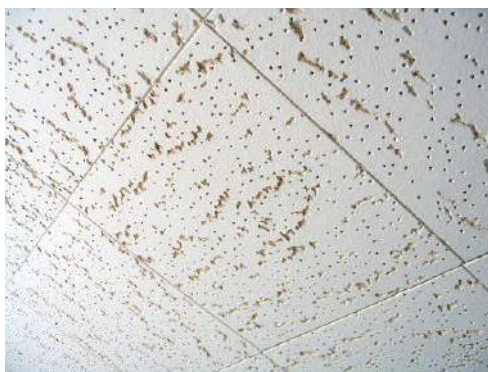
Asbestos containing ceiling tiles
