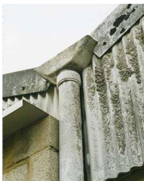
Asbestos cement downpipe, hopper and profile sheet
