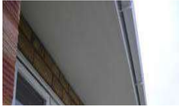
Pieces of Asbestos Insulating Board (AIB)
