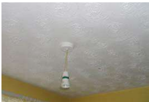
Asbestos textured coating
