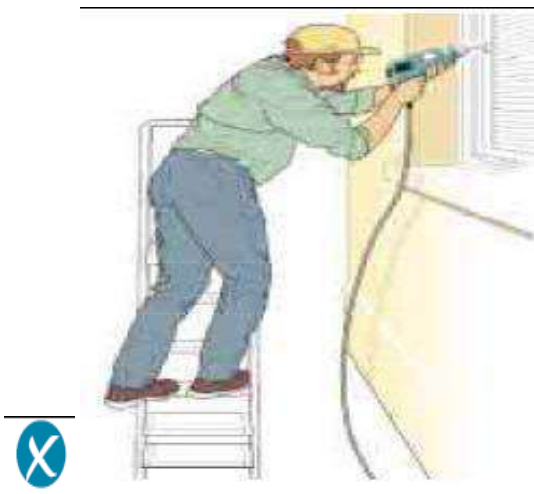
Incorrect – steps side on to work activity
