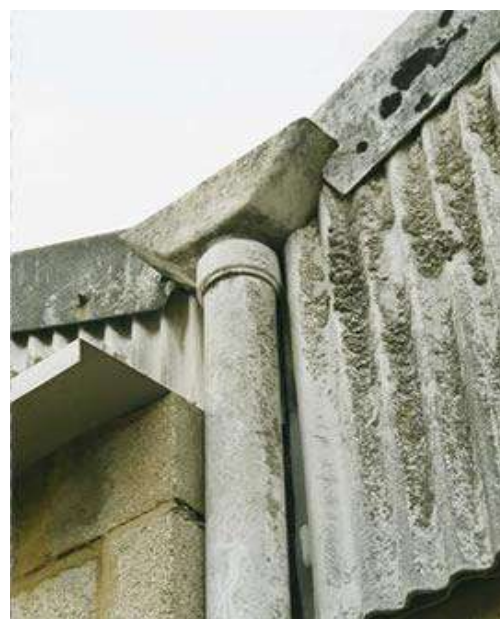
Asbestos cement downpipe, hopper and profile sheet
