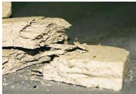
Pieces of Asbestos Insulating Board (AIB)
