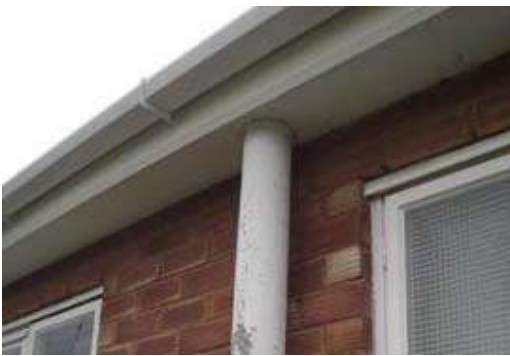
Asbestos cement drainage pipe (downpipe)
